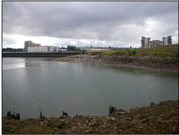
Photograph 4: West harbour (internal).
