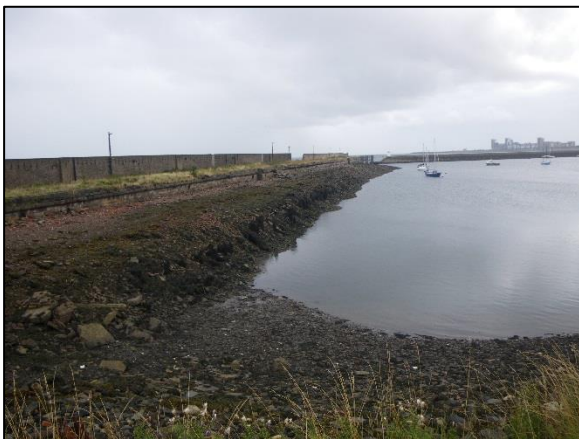
Photograph 5: North harbour wall (internal).
