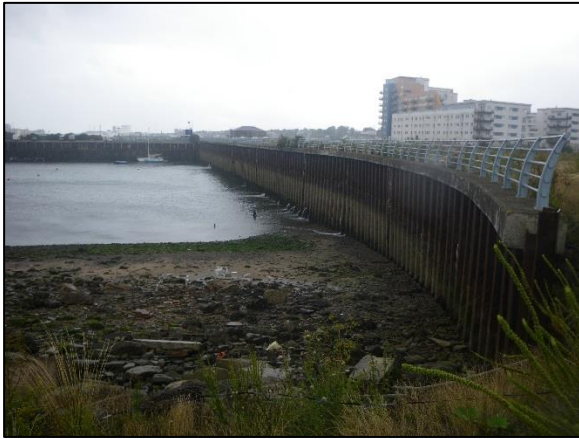
Photograph 3: South harbour wall (internal).
