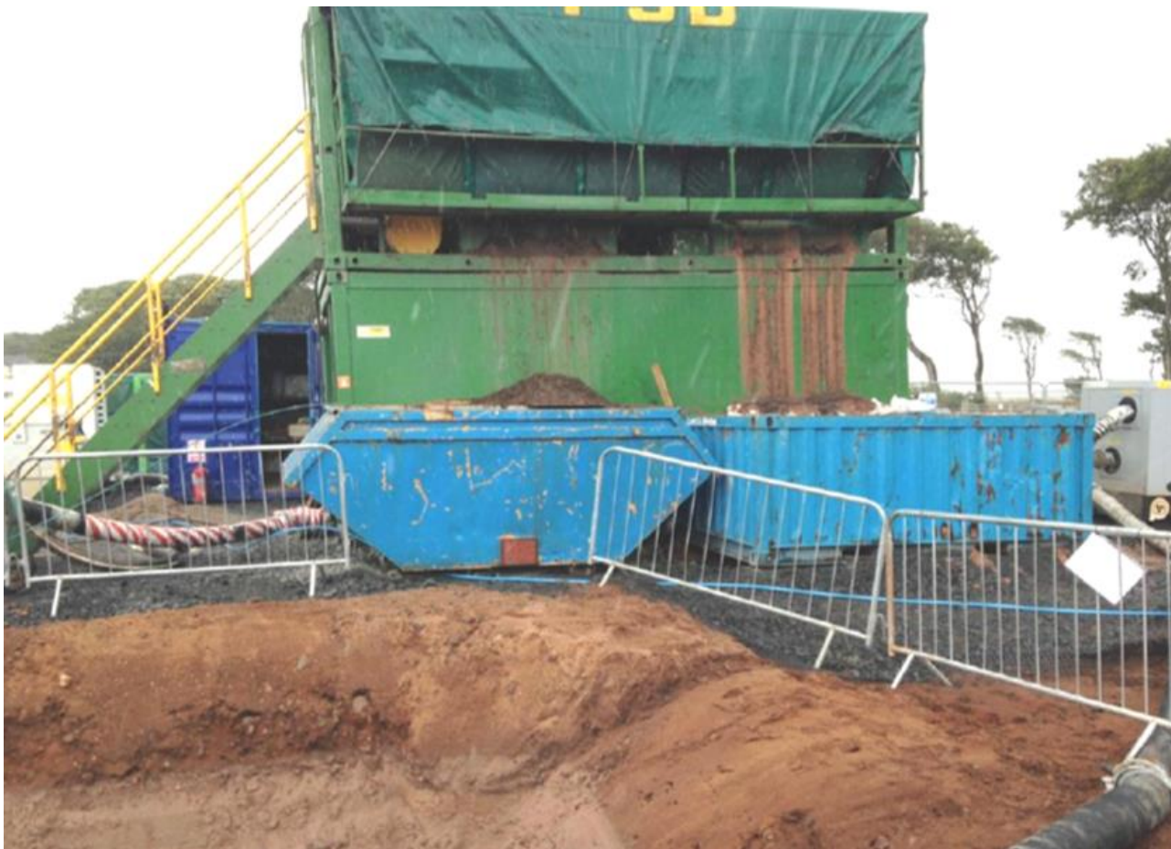
Figure 5.2: Example Drilling Fluid Recycling Unit
